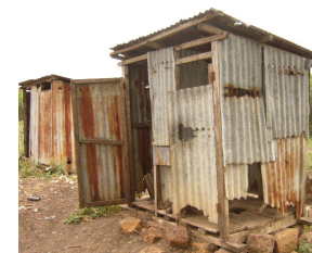
Poor sanitation: A decaying pit latrine that is still used in Makongeni Estate – Homa Bay (Kenya). Photo: UCSD
