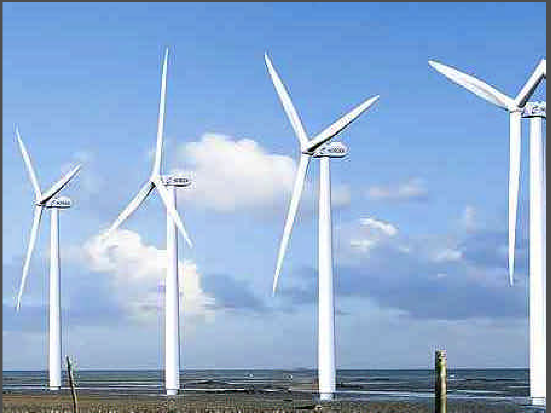
Photo: Courtesy of Brown Energy Systems
