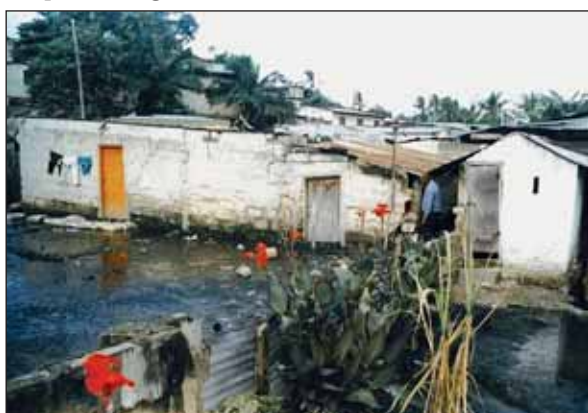
A sinking house in Mwananyamala, Kisiwani, Dar-es-Salaam, Tanzania.
