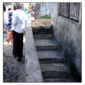
Figure 3. Flood protection wall around a house in Tandale
