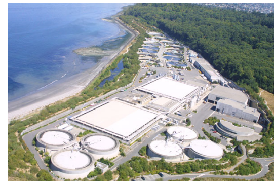
West Point Treatment Plant Seattle, Washington
