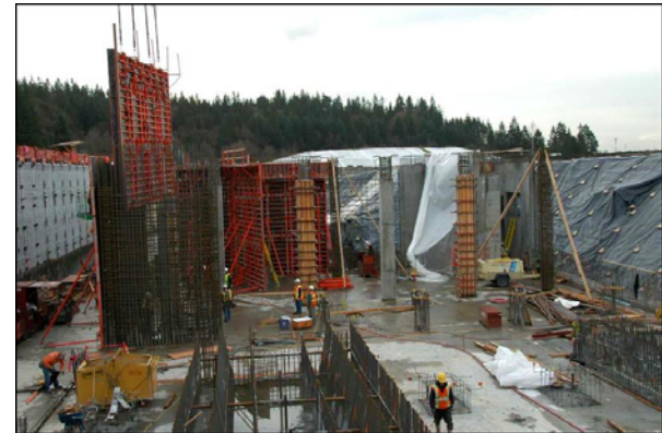
Brightwater Treatment Plant construction
