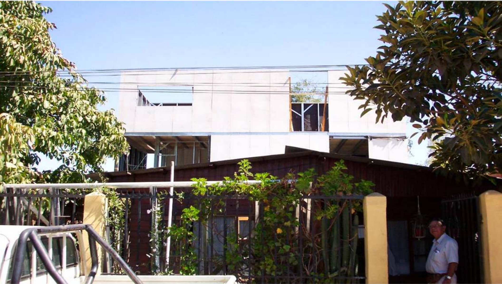
The house from the street
