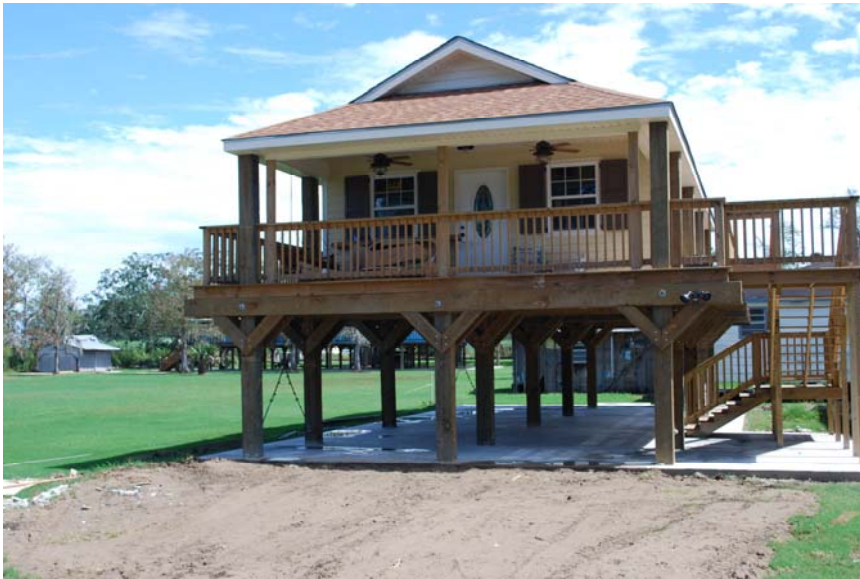
Louisiana Lift House
