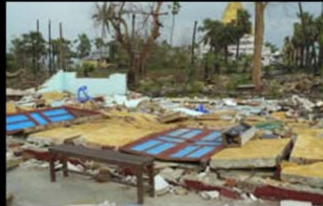
Another building at the orphanage is totally destroyed
