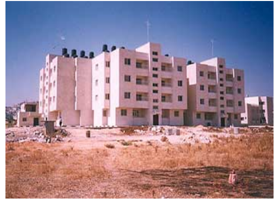
Senger Housing Project - Hebron
