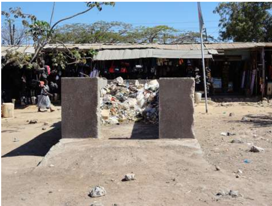
Figure 6.1: Solid waste collection bay at the main market in Sengerema, Tanzania
