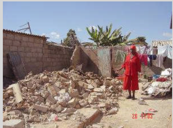
Backyard demolition in Chitingwiza, Harare.
