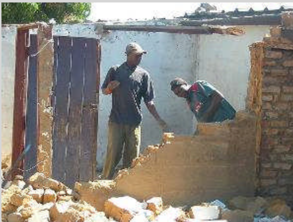
Owners demolishing their own house in Epworth, Harare.
