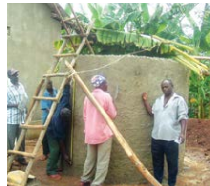
Construction of the rainwater harvesting tank. © UN-Habitat
