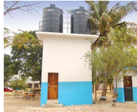
Newly constructed water storage facilities and a panel house. © UN-Habitat
