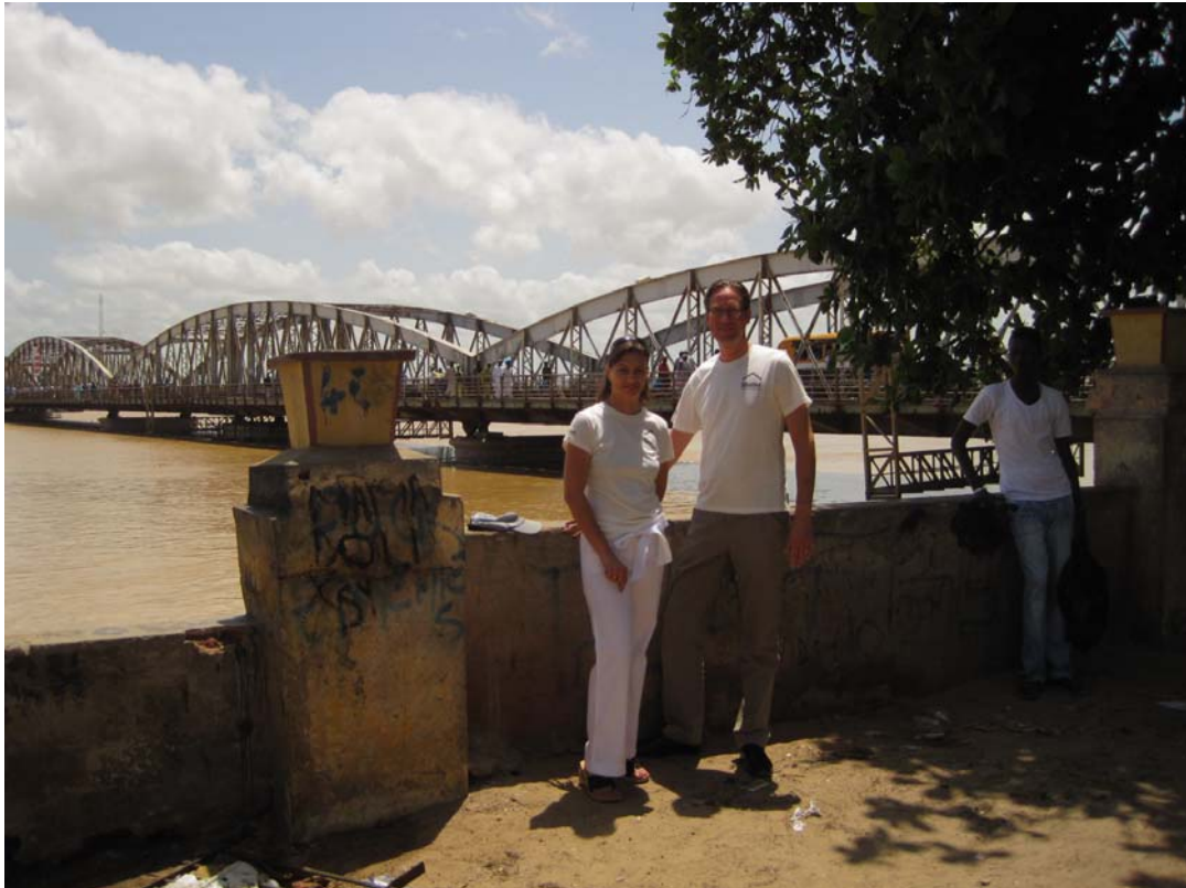
Photo 29: The famous bridge connecting the main island of St. Louis with the island of Sor (bridge was under reconstruction)
