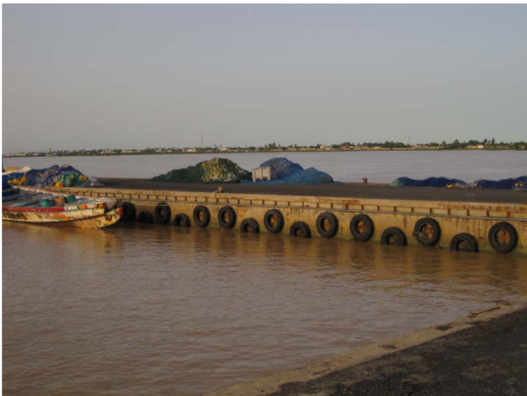
Photo 14: the locally called "Polish Port" is hardly used by the fishermen because the quays are too high for their boats.
