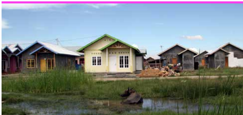
Section of newly constructed houses after Tsunami in Banda Aceh, Indonesia ©UN-Habitat
