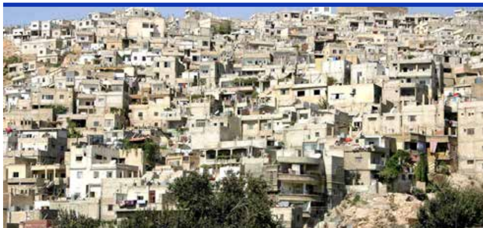
A view of an illegal neighborhood on the north-east edge of Damascus, Syria. Up to 40% of construction in the city is done without approved official plans © Hugh Macleod/IRIN.
